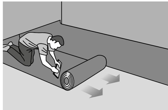
It's important to use the cork press when you gradually roll out the sheets onto the adhesive. In this way, you will avoid catching air under the sheets that may cause blisters later on.
